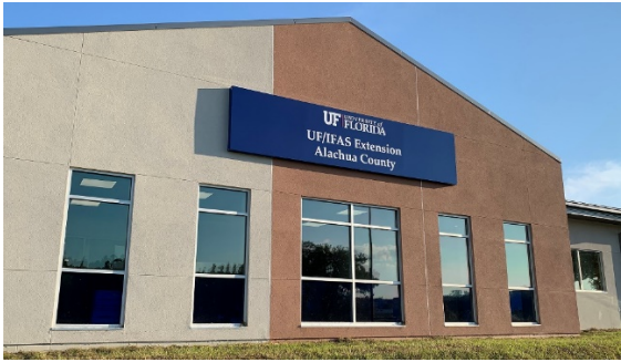
Completion of the new UF/IFAS Extension Alachua County and Ag Auditorium Building
